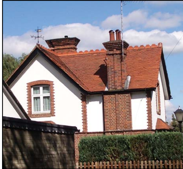
Detailing to Island cottage with the prominence of the brick quoin, window detailing and the attractive chimneys
