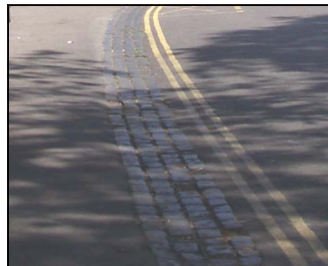
Kerb detailing in small stone blocks
