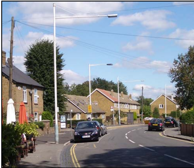
Street lighting inappropriate to Conservation Area
