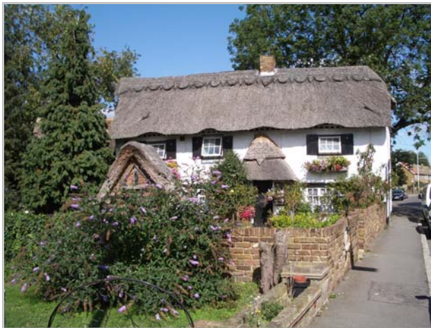
View looking north east towards 532 Bath Road
