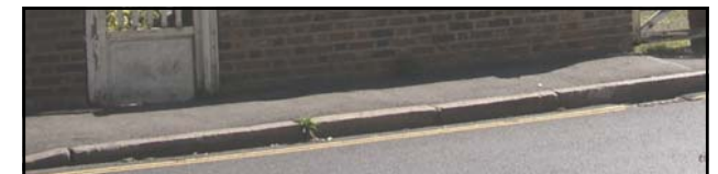
Kerb detailing in long stone blocks
