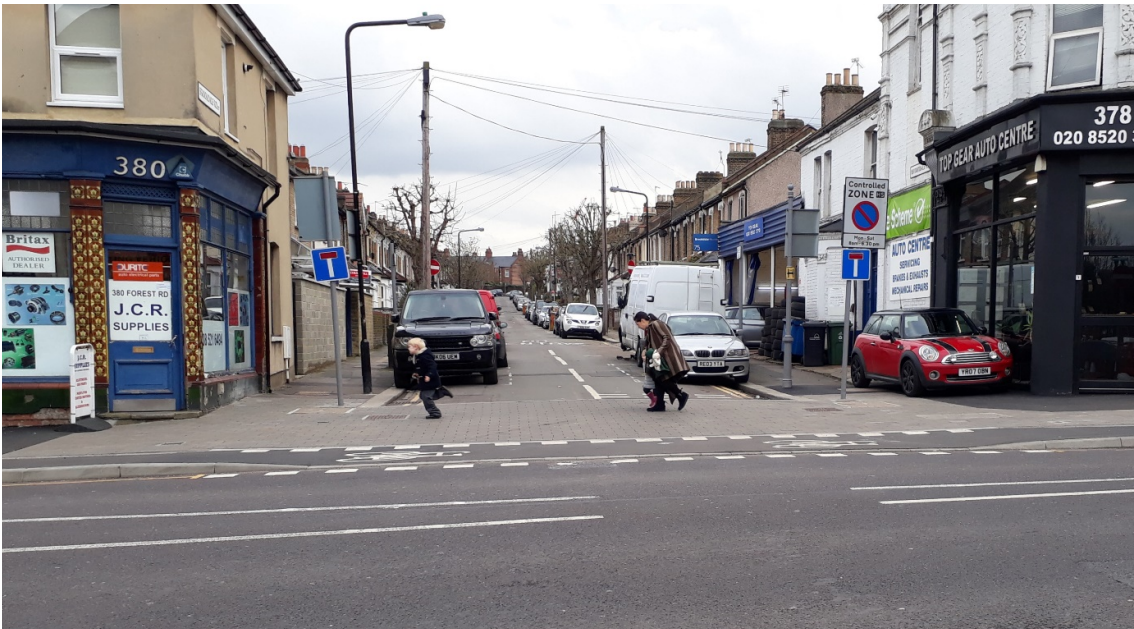
Figure 23: Continuous footway offering design priority to pedestrians.
