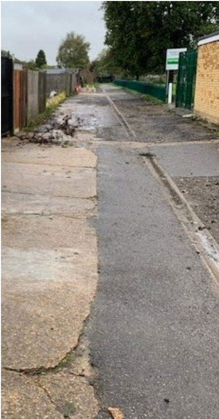
Skipton Drive service road leading to Bourne Farm Playing Field – Before
