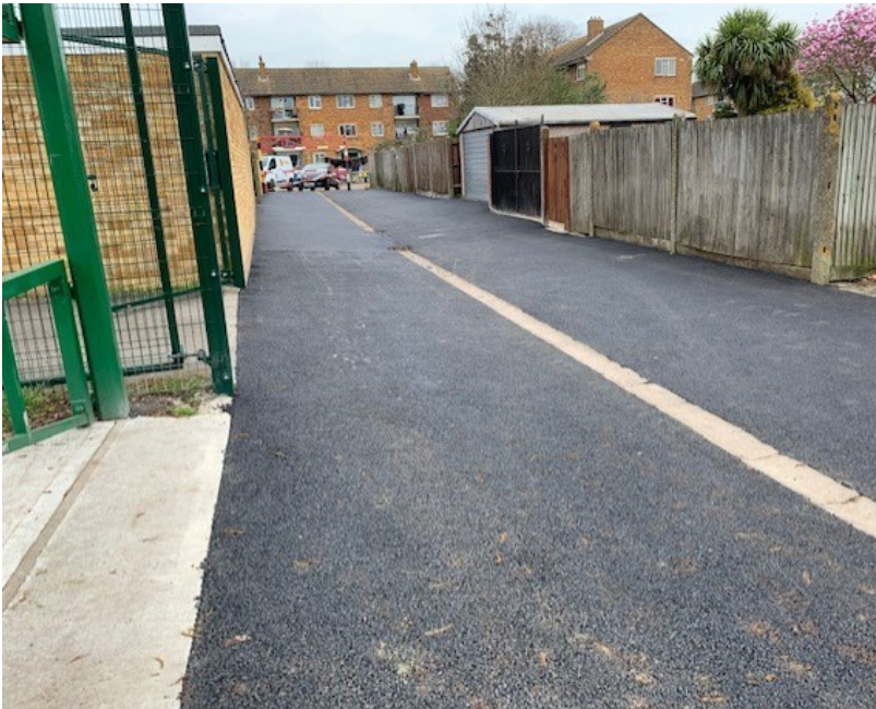
Skipton Drive service road leading to Bourne Farm Playing Field – After
