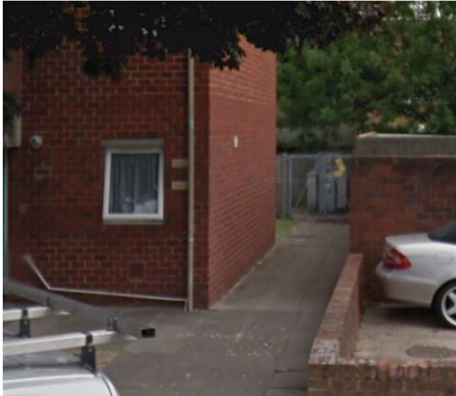
Albion Road - Before
