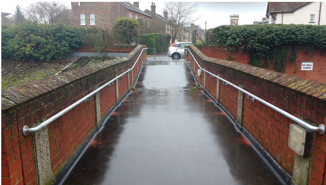
Whitehall Road safety rail installation – After
